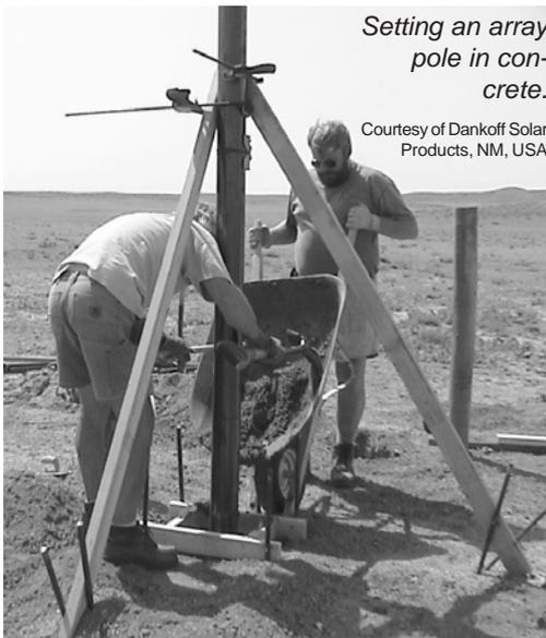
*Setting an array pole in concrete.*
