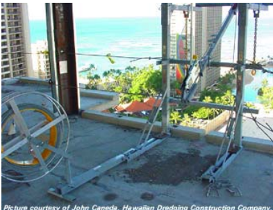
Picture courtesy of John Caneda, Hawaiian Dredging Construction Company.
