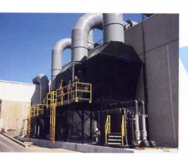
This version of the horizontal system is available with ANSI or vertical pump systems. The system is not limited in size by the type of pump available. Both large capacity ANSI and vertical pumps are available in this version. Standard pump materials of construction for both versions include FRP, polypropylene and stainless steel.
